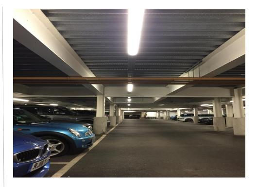
The savings calculations for the client are based on the wattage reduction from the existing T8 twin fittings dropping down to a 35w LED offering, but there is the maintenance of the old lights to take into account here too. Many companies just base the investment on wattage for wattage savings, but in many cases the time spent by staff assessing the failed lights, ordering new tubes and fittings as well as the time to refit these items all adds up.
